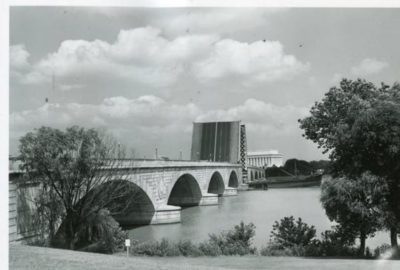
The Memorial Bridge was built with a drawbridge originally, but this bascule is now being replaced by a joint DDOT and Federal Project.
